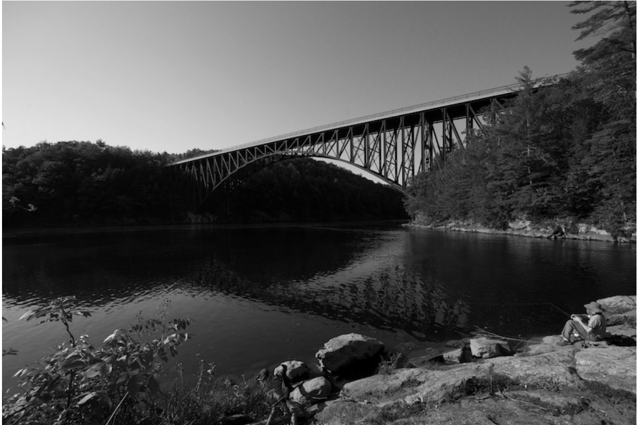
French King Bridge Over Connecticut River - Erving
